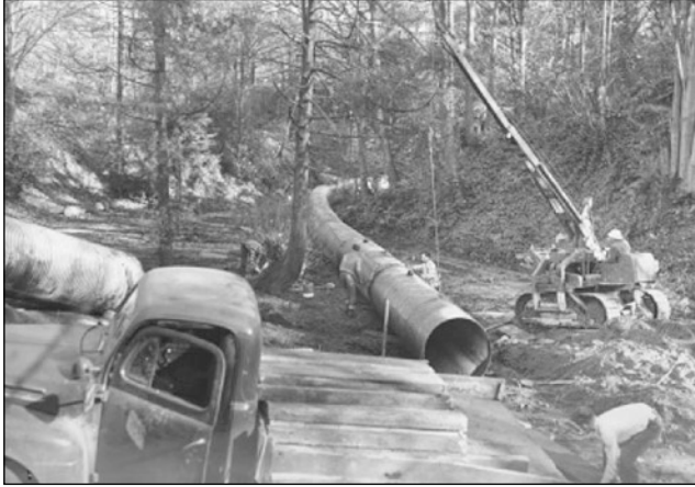
34. Temporary Sewer running through the park.
