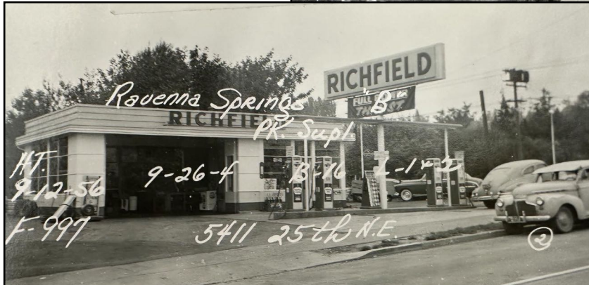
Corner Gas Station, ca. 1975
