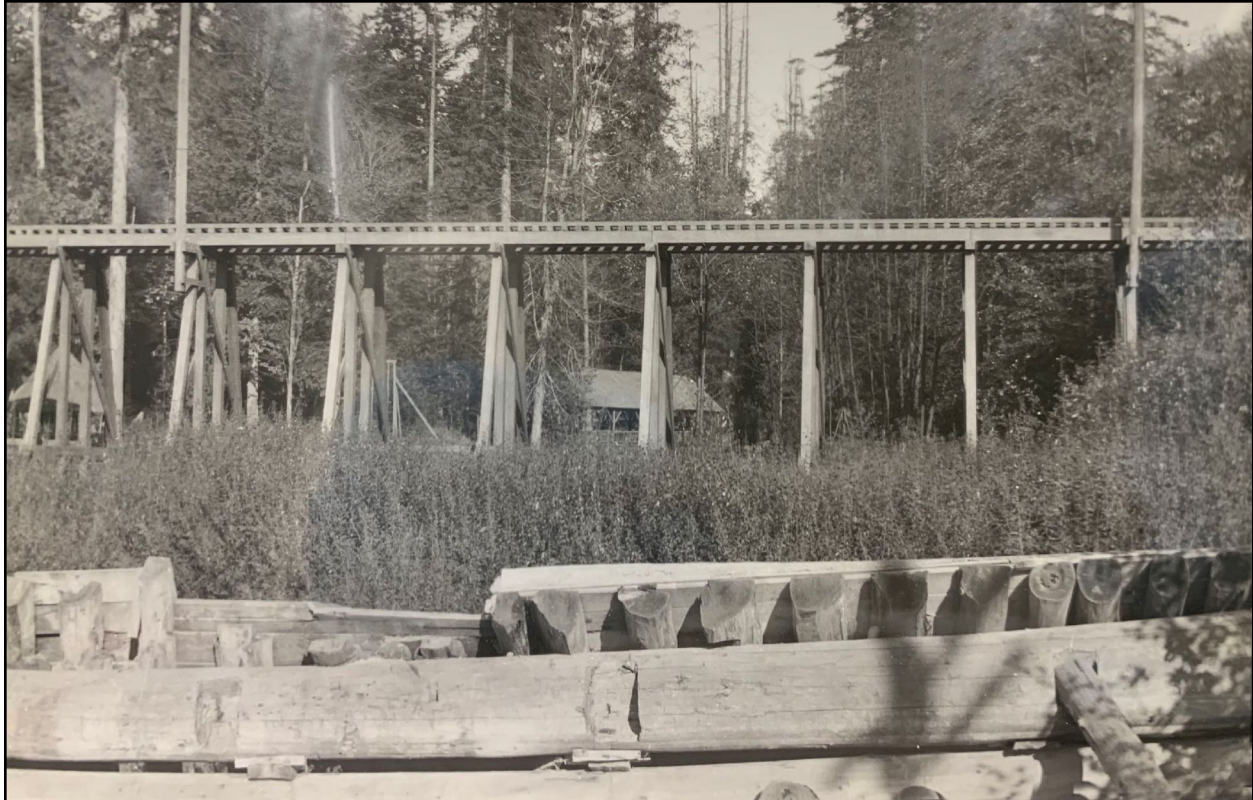
Streetcar Trestle Across the Former Pond. Breached Dam in Front
