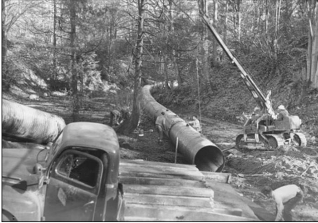
37. Temporary Sewer running through the park.
