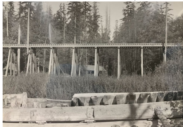
24. Streetcar Trestle, 1910. See Covered Bridge in distance.
