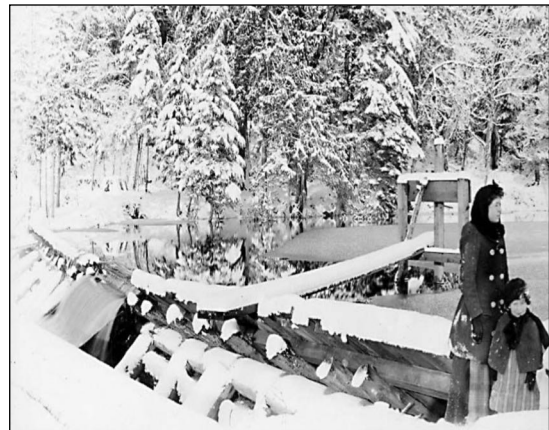
20. Wooden dam, ca. 1893.
