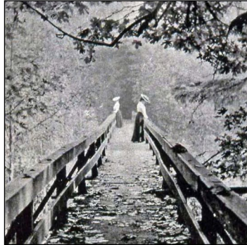
8. Ravenna Park Bridge, ca. 1909
